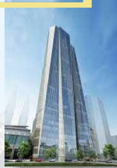
Permata Sapura Tower
